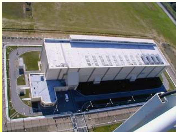
Interim Storage Facility Emsland
