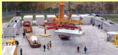
storage facility at Neckarwestheim
