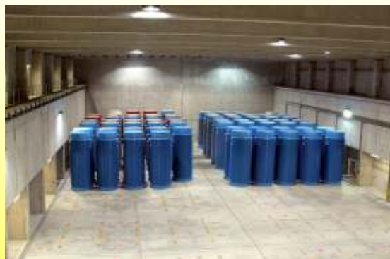
Gorleben interim storage facility, the storage facility for vitrified waste from reprocessing
